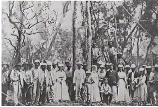
Figure 2 – Erecting the first telegraph pole for the Overland Telegraph Line in Darwin in 1870
